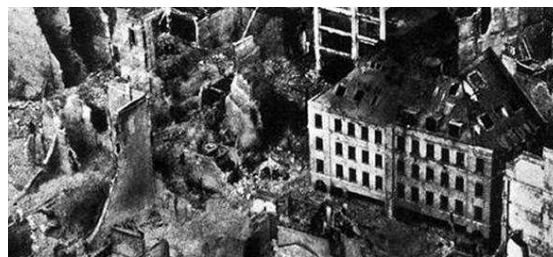
Destroyed and damaged London houses after the hard attack on 10 th May 1940.
